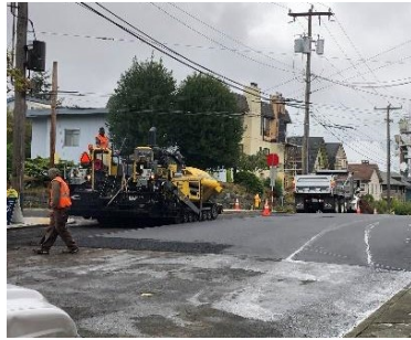
A road is resurfaced.
