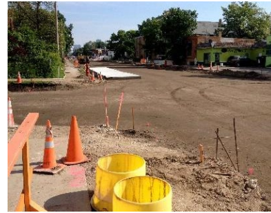
A road is reconstructed.
