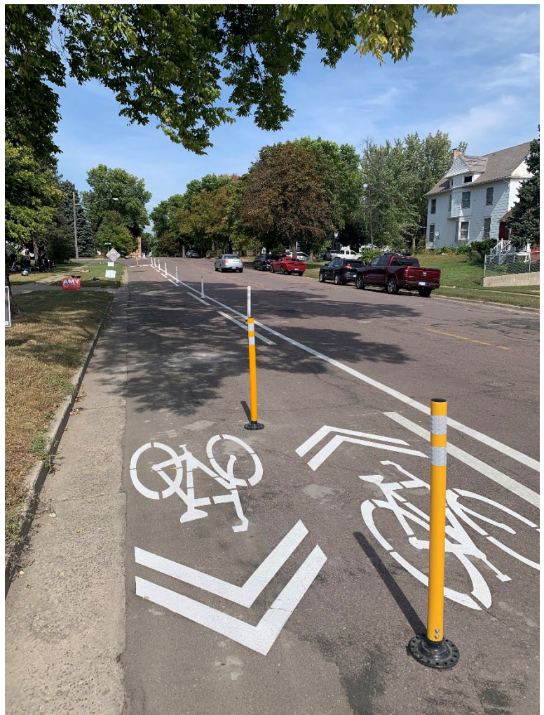
Figure 4: Installed Demonstration Project
